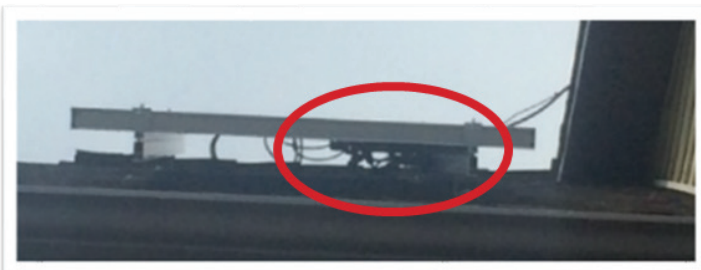
Photo 8: Source circuit conductors in contact with roof: NEC 338.10
