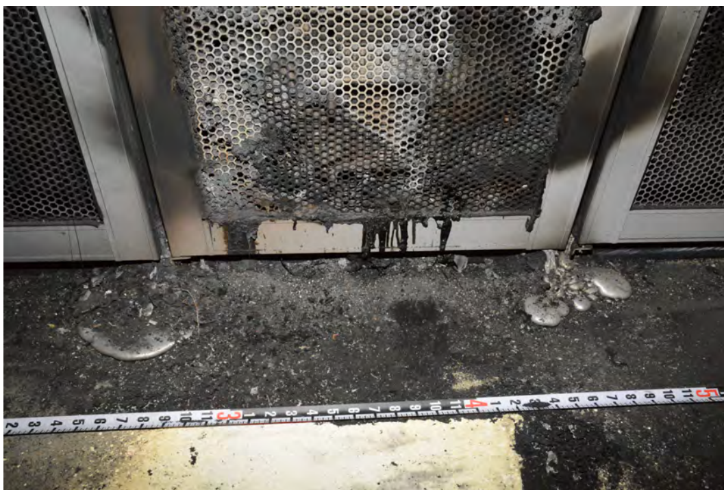
Figure A.1: Photograph taken during decommissioning of the ESS shows a pool of solidified aluminum on the floor in front of Rack 15 [11].
